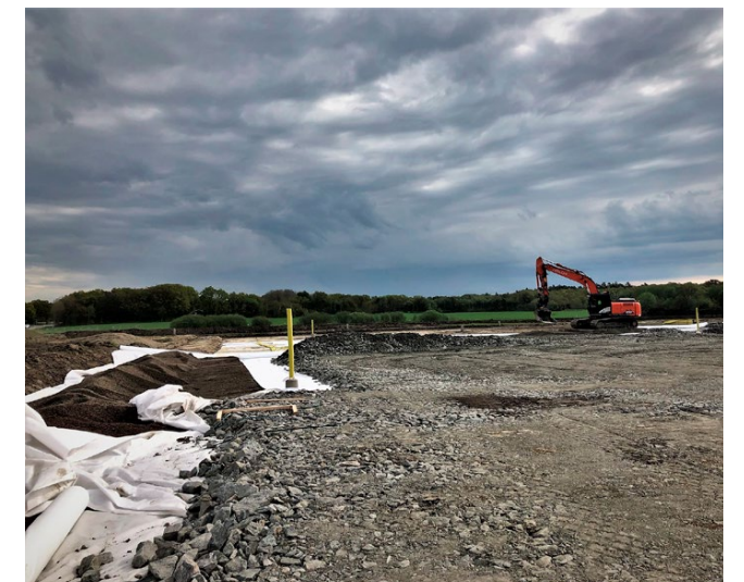
A solid foundation on the soft soil that will reduce the risk for settlements.
