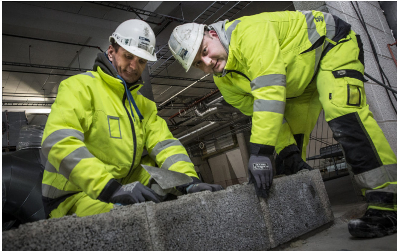
The new blocks with tongue-and-groove made it easier for Tomas Urban and Roman Lewandowski to achieve a good result.
